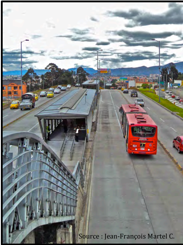
Figure 8 : Station de TransMilenio
